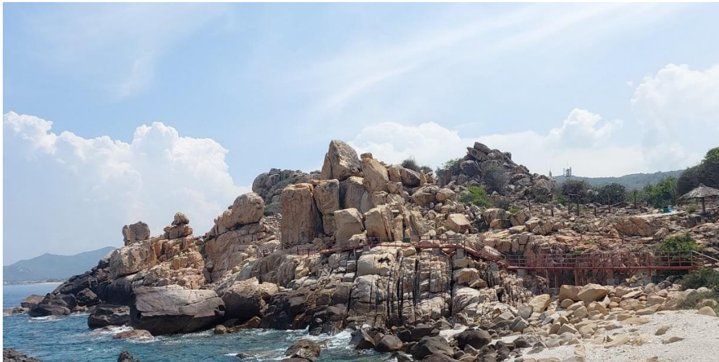
Fig. 1. Tectonic cliff coast resulted in a characteristic balanced rock terrain in phases 2 and 3, as classified by Geikie (Twidale and Romani, 2005). (Source: Hoang et al., 2021)
