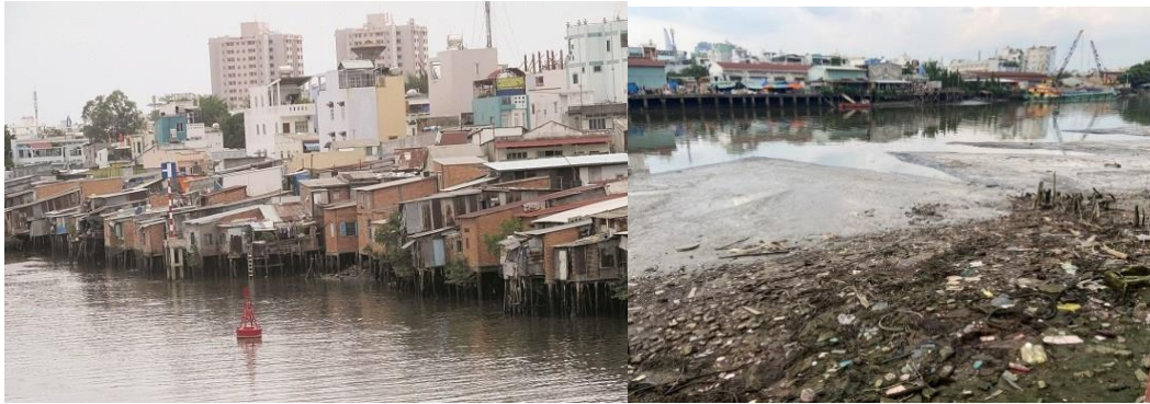
Fig. 2. Houses encroach on the canal, discharging waste water directly into the canal.
